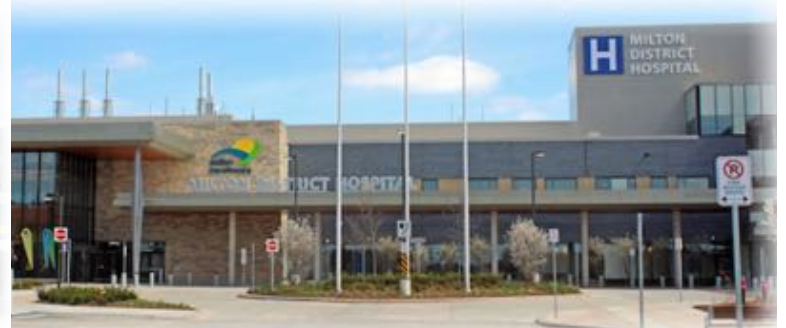
Milton District Hospital
